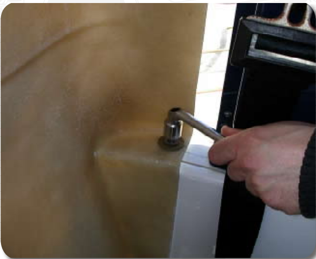
7/ Install the element lateral to the panel, put a mark for the drilling.
